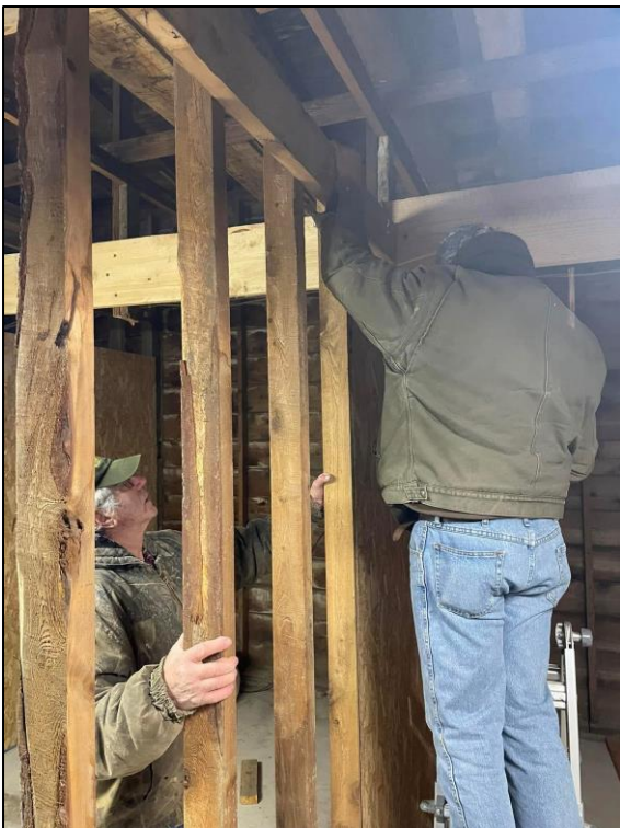
Supporting structure also serving as theme room wall studding.
