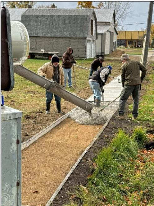
With upfront preparation complete, the cement is being poured.
