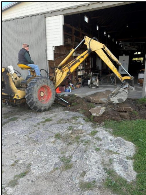
Breaking up and removing the old concrete.
