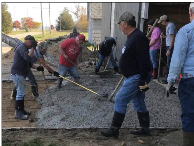
The concrete is poured, shoveled pushed and leveled.
