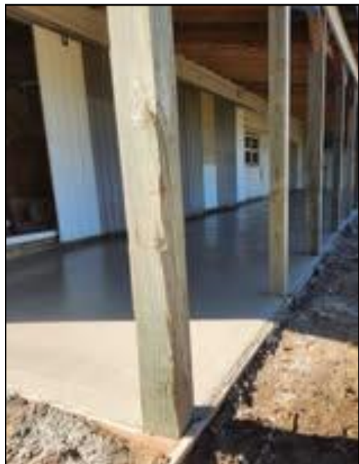
Concrete floor laid under the entire overhang.
