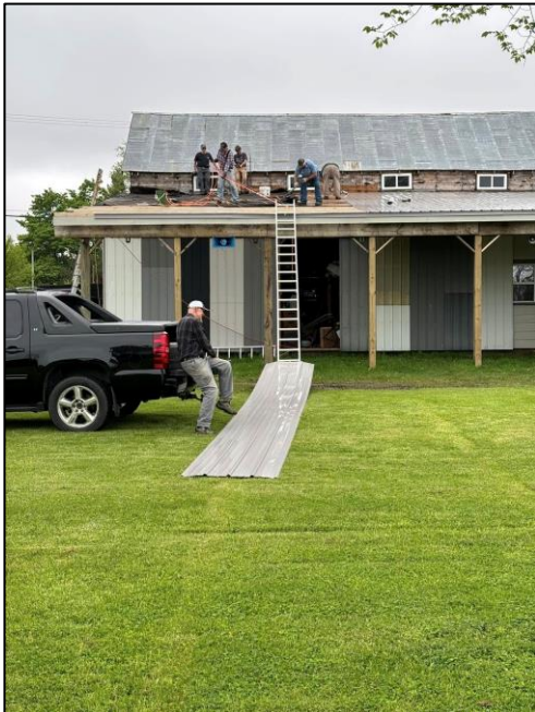
Roof boards and metal roofing installed. Structure nearly complete.
