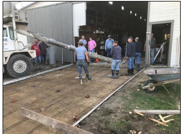
Framing, Leveling, sand filling, laying out the reinforcing rods, all complex stuff, and most likely done by the same volunteers that did the roof and wired the building.
