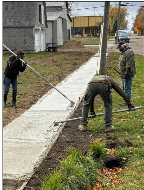
Final leveling and smoothing and we're nearly complete.
