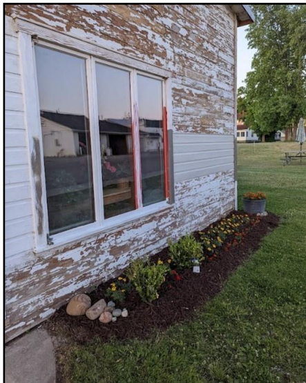
Front face of our building being blasted, scraped and readied for paint.
